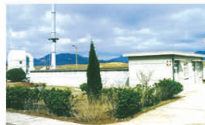
Gallery Propane Buring Station
