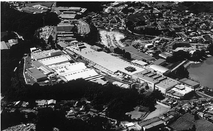
KITZ Nagasaka Plant, Japan
