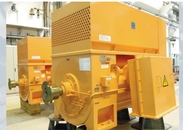
Pump drive High-voltage asynchronous motor with squirrel-cage rotor 800 kW / 11,000 V / 994 rpm
