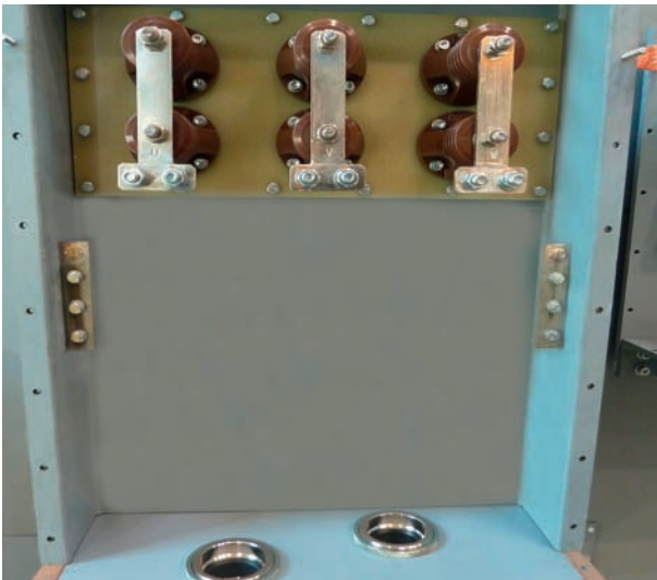
Example of a rotor junction box
